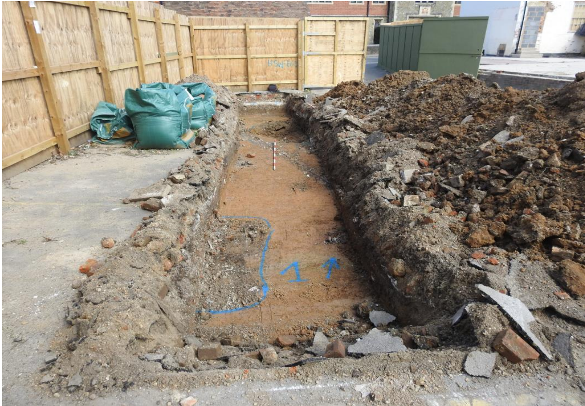
Plate 3: Trench 1, looking north with two-metre scale.
